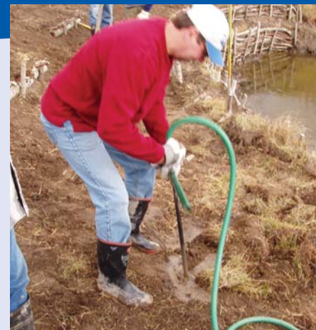
The initial row of live poles for wattle fences are placed near the water's edge. These poles are usually larger in diameter than the poles placed horizontally behind this row. Poles should be at least 80% underground as being demonstrated here.
