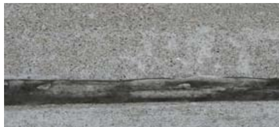
This hardscape crack, filled-in with soil, has become the perfect planter for weeds. (above) Caulking prevents hardscape cracks from filling in with soil. (below)
