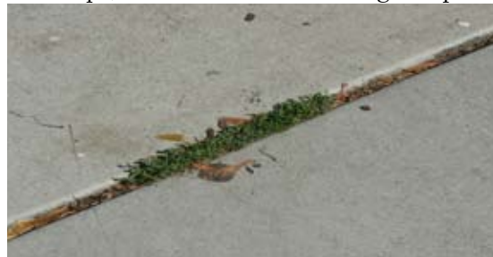
This hardscape crack, filled-in with soil, has become the perfect planter for weeds. (above) Caulking prevents hardscape cracks from filling in with soil. (below)
