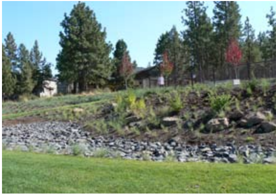
A bioswale (rocky area), installed in the newly constructed Quail Park in Bend.
