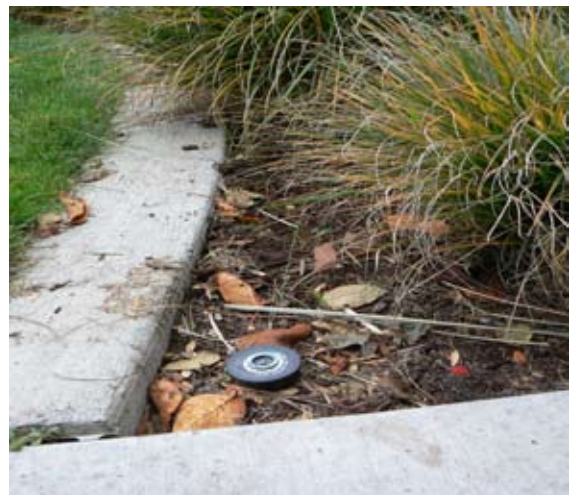
A border strip in Alki Park in West Seattle is elevated above the bed to block weeds from entering.
