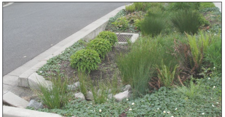
A curb bump-out and rain garden in Portland, OR. Photo: DC Green Infrastructure
