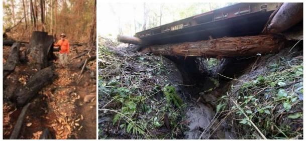
At Doubleduke (Pugh 2010b) we found two poorly constructed creek crossings without implementation of soil stabilisation measures that resulted in significant mobilisation of sediments into both streams (Breaches EPL J45, J46, J52, FL 8.4.1.(a), 8.4.2.(b), 8.4.3.(b)). Forests NSW subsequently implemented erosion mitigation works at both crossings, though Fisheries NSW were not informed of our complaint.
