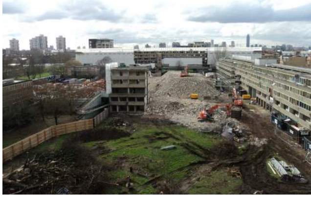
View from the 8th floor showing the ongoing demolition
