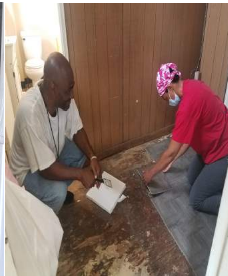
Ty & Shelley laying tile
