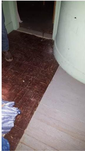
5. Image showing 9" X 9" floor tile (and mastic), mint paint, and gray paint on 2<sup>nd</sup> floor.
