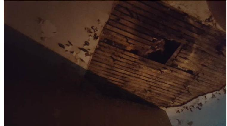
2. Image showing plaster, vermiculite, and white paint of second floor ceiling.
