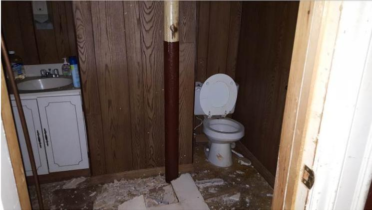
1. Image showing bead board (and glue), sink lining, basecoat (and mastic), beige/peach paint, and burgundy paint on 2<sup>nd</sup> floor.
