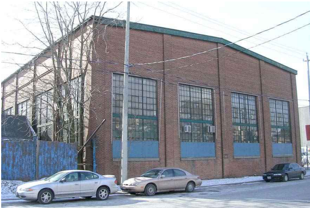
Image 1: 185 Eastern Avenue - Foundry B80036
