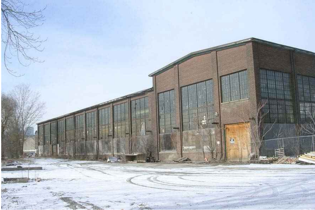
Image 4: 153 Eastern Avenue – Machine Shop B80086
