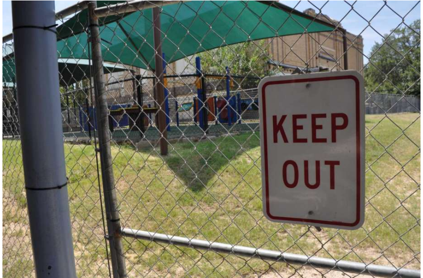
Children are fenced off from a playground at Beacon Hill Academy because the building is considered unsafe. Parents want a solution. Photo: Josh Brodesky /Express-News
