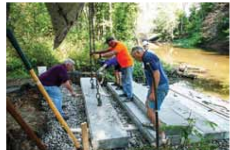
Construction of the new Byron Canoe and Kayak Launch
