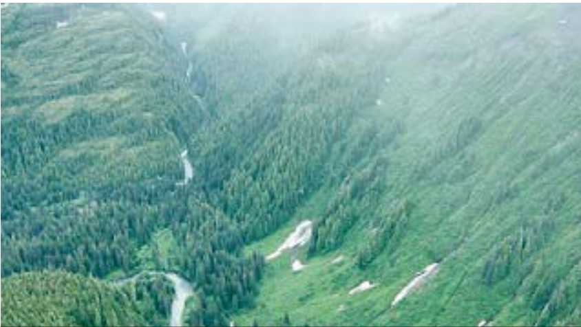
Logging decreases slope stability, but even old-growth forests succumb to gravity. This old-growth forest has been cleared by debris flows and avalanches.
