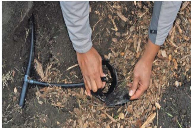
*Adjusting flow by rotating the tees. Ball valves can be added to the ends of small tubes, if necessary. Photo: David Glover.*
