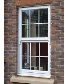
Sash or hung windows in poor repair may pose a risk. If the the sash is missing the chord or weights that counterbalance the sash window, the window may drop unexpectedly, potentially hitting a person or shattering glass. Always open sash windows with care and be prepared to prop window open if it doesn't stay open itself.
