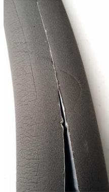
The hot water outlet pipe from your hot water cylinder should be insulated, at least for the first 2 m or as far as can be accessed. If the tank and pipework are inside or under the house we will supply Armaflex flexible pipe insulation. This is presplit with adhesive. Simply place over pipe and remove adhesive covers and pipe will seal.
