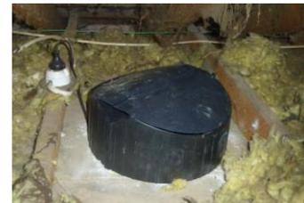
Ceiling exhaust fans and combination light/heater/exhaust units (e.g. IXL Tastics) are problematic as they are a large hole in the ceiling, drawing heat from inside the building into the colder ceiling cavity. The hottest air accumulates in the ceiling, so exhausts allow considerable amounts of heat to escape into the ceiling cavity.
