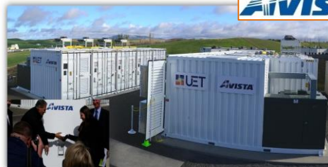
1 MW / 3.2 MWh UET vanadium-flow battery – Pullman, WA
