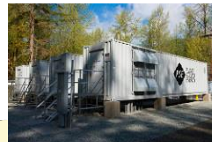
2 MW / 4.4 MWh lithium-ion/phosphate battery – Glacier, WA
