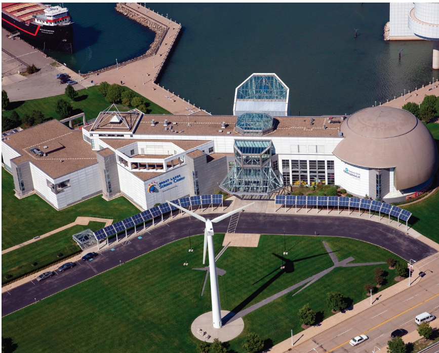
Onshore wind turbine w/ peak output of 225KW at wind speeds of 31 mph. Solar array canopy producing an annual average of 100KWh/day at the Great Lakes Science Center, Cleveland.
