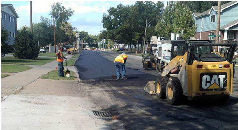
Manhattan, KS, street repairs ( https://cityofmhk.com/2584/Street-Maintenance-Sales-Tax )
