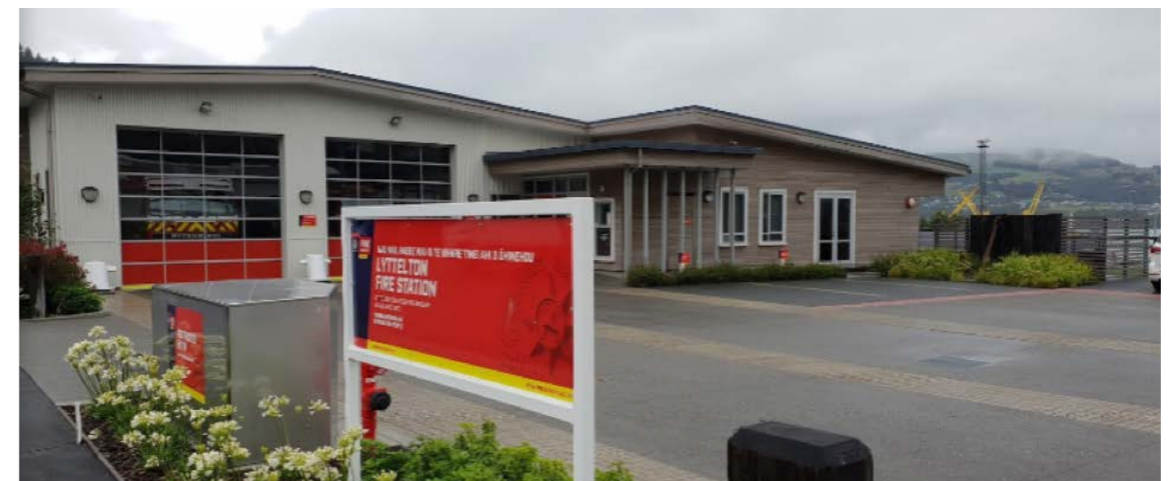
LYTTELTON URBAN VOLUNTEER FIRE STATION BUILD. FLOOR AREA 497 SQM. COST $3.85 MILLION – 2017
