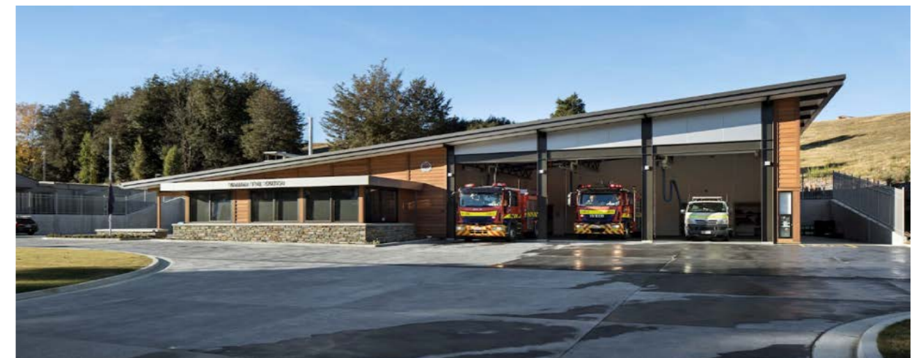
WANAKA URBAN VOLUNTEER FIRE STATION BUILD. FLOOR AREA 585 SQM. COST $3.96 MILLION – 2017
