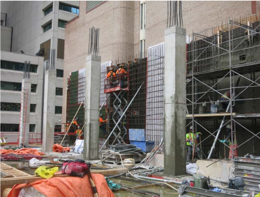
North-west view from the second floor, showing the concrete columns that will eventually support the floor above. In the background, the north wall of the courthouse is taking shape. (November 2019)
