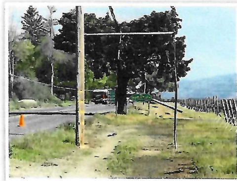
When a power pole is hit, there are additional risks of fire and electrocution from downed wires.
