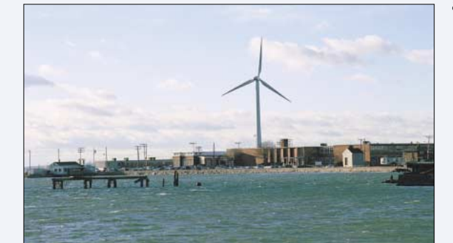
The citizens of Hull, Massachusetts installed the first commercial-scale municipal wind turbine on the east coast in December 2001. Their 660 kW turbine has allowed the municipal light plant to discontinue billing for powering the town's streetlights and traffic signals, saving the Hull's 11,000 citizens more than $50,000 per year. Hull is now considering installing a second, much larger turbine along side Hull Wind 1 on Windmill Point.
