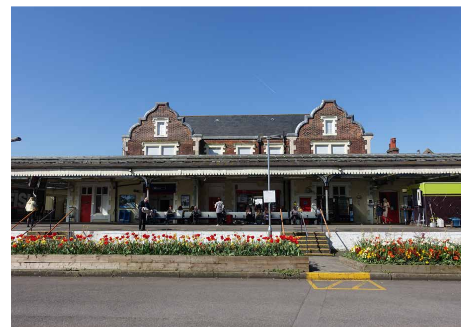
Entrance into station from existing car park
