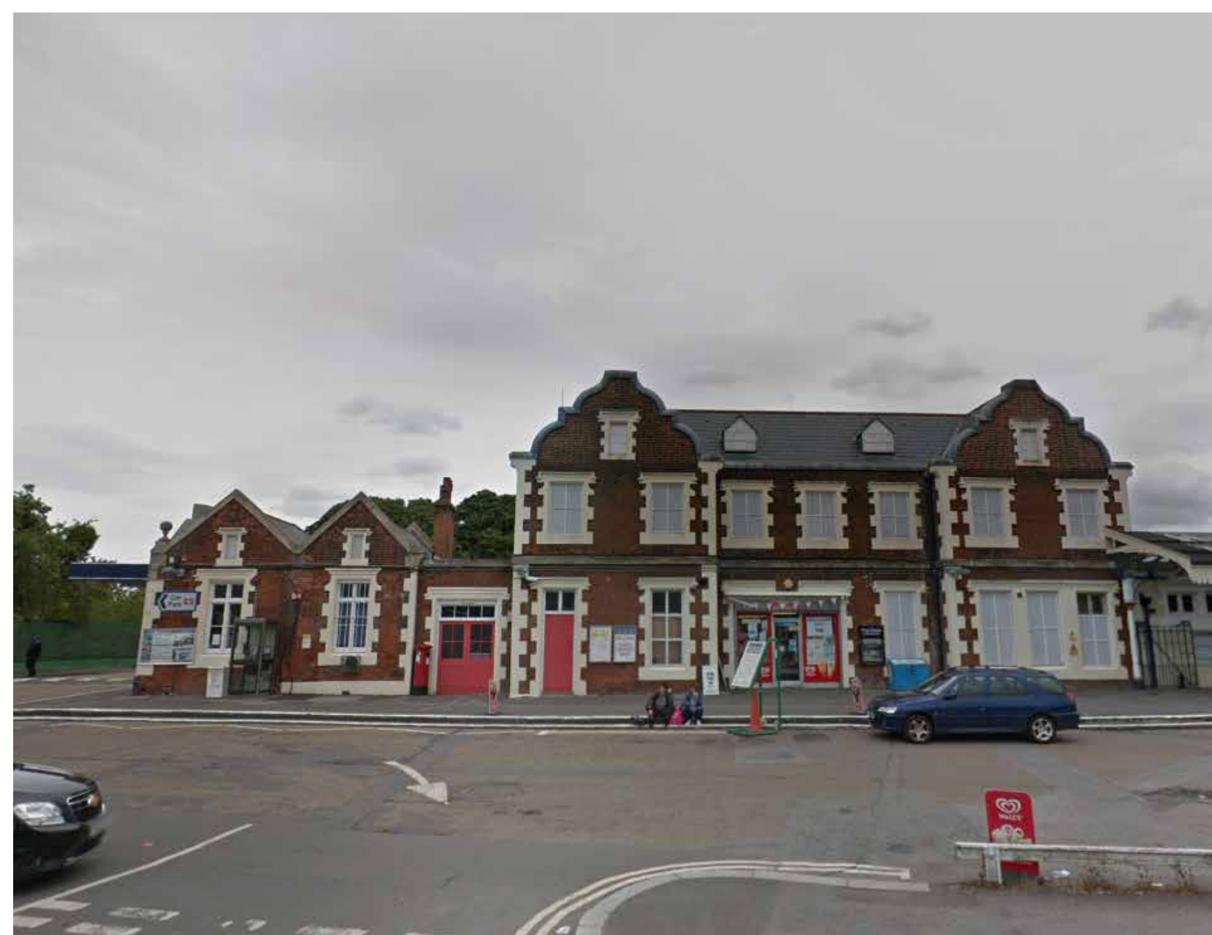
Existing taxi / bus drop off area outside station entrance
